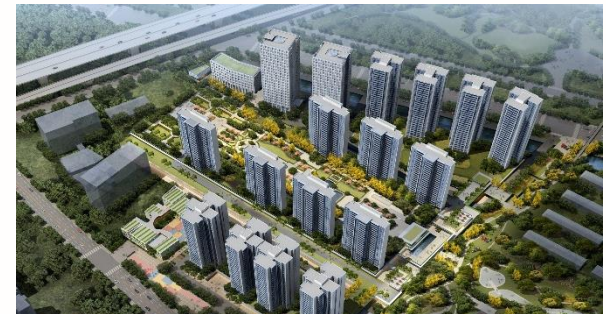
Foshan Metro Depot Cover Project
